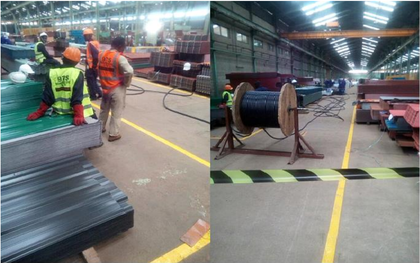
97's Engineering Roofings Factory works: Cable Laying and installations
