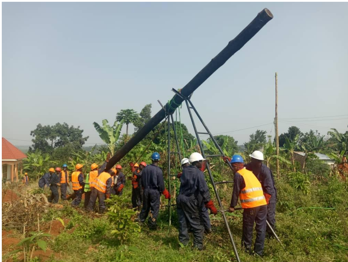
Power line Diversion a long Busega-Mpigi Expressway UNRA Road Project
