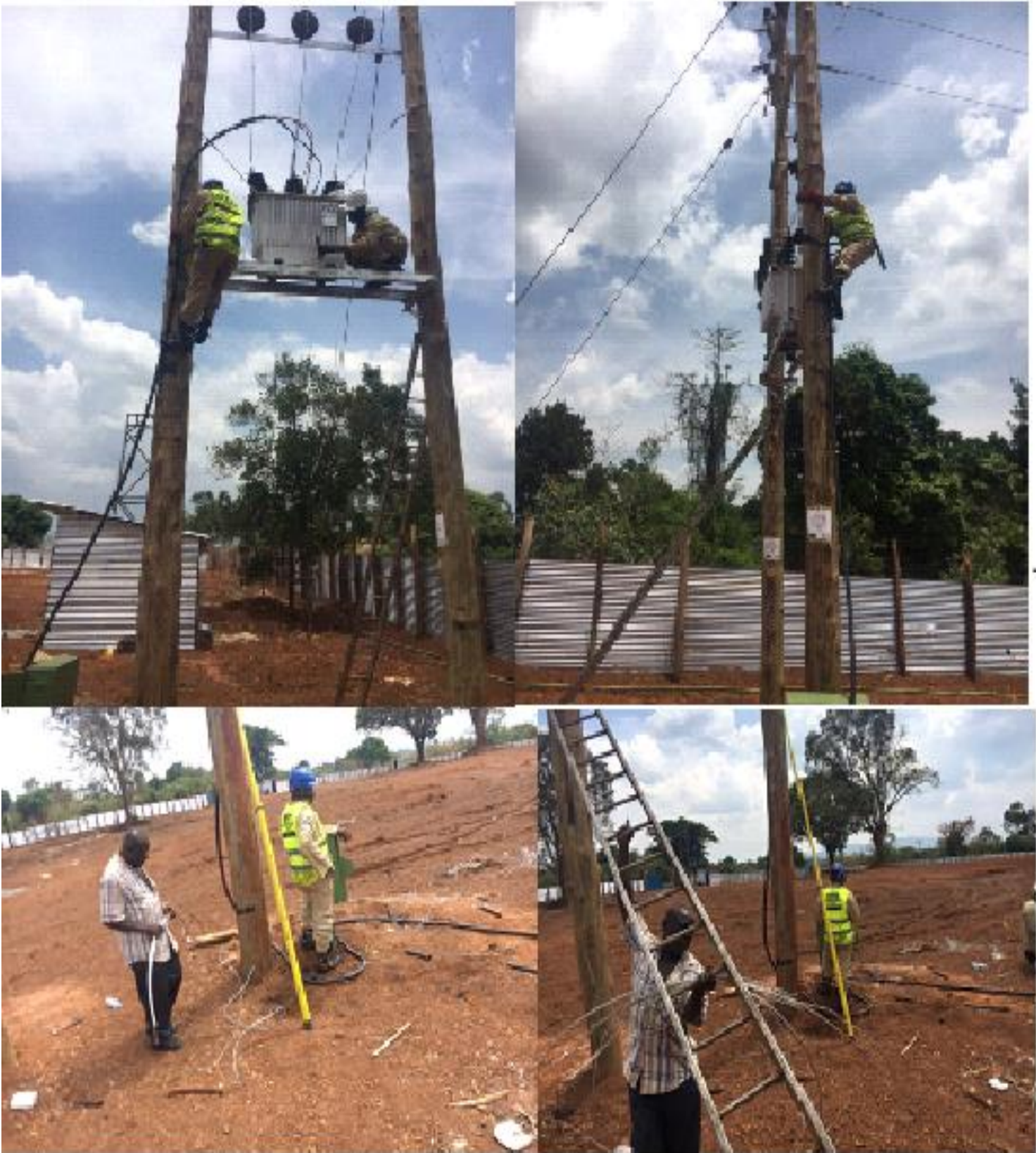
97s Engineering Hoima project: Construction of Distribution Power Line
